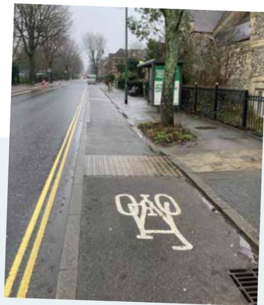
**Protected cycle lane, separated from both the road and the pavement** (Old Shoreham Road)
